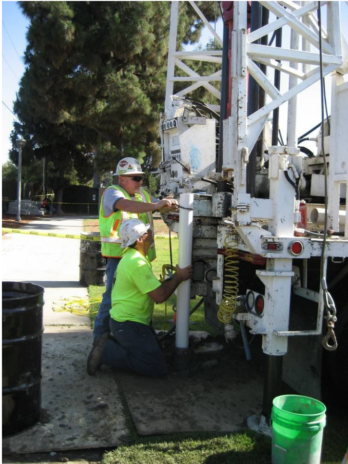
Well installation of GMW-62
